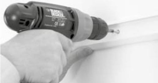
Put the top track up with one screw and tighten it enough to hold the top track against the wall.
