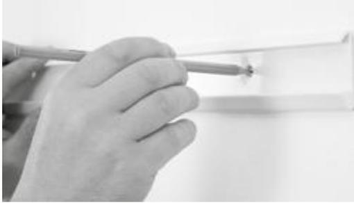
Place top track at desired height, mark one hole in the middle, and take the top track down. It is usually placed at ceiling or door height, but may be placed at any height.
