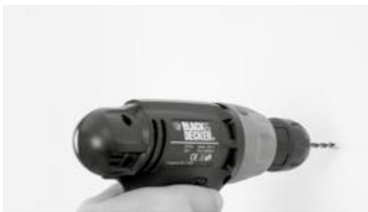
Begin drilling the marked hole with a 1/8" / 3mm drill bit. If you hit wood, continue drilling the entire length of the bit. If you hit the hollow part of the wall, enlarge the hole with a 3/8" / 10mm drill bit for the hollow wall anchors.
