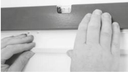
To keep the top track level while you mark **all of** the holes, place a level on the top of the top track and adjust it as required.
